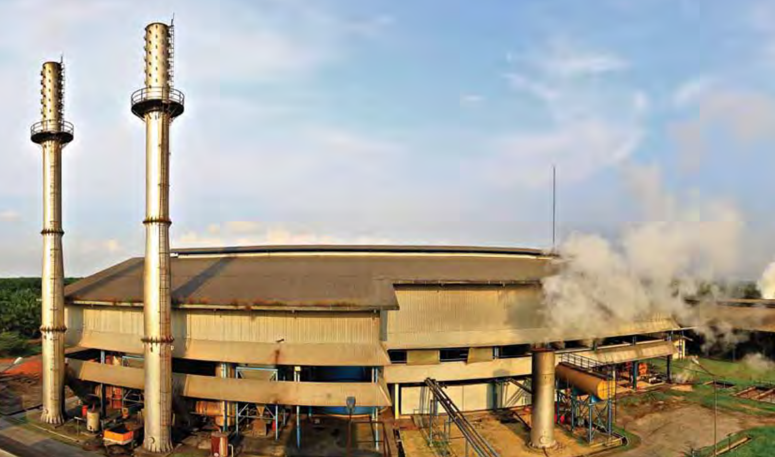
Pabrik Kelapa Sawit Unit Sumut 1 Palm Oil Plant Unit 1 North Sumatra
